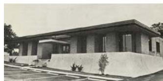
As the association grew, it constructed a new building in 1969 on I-35 in Austin.
